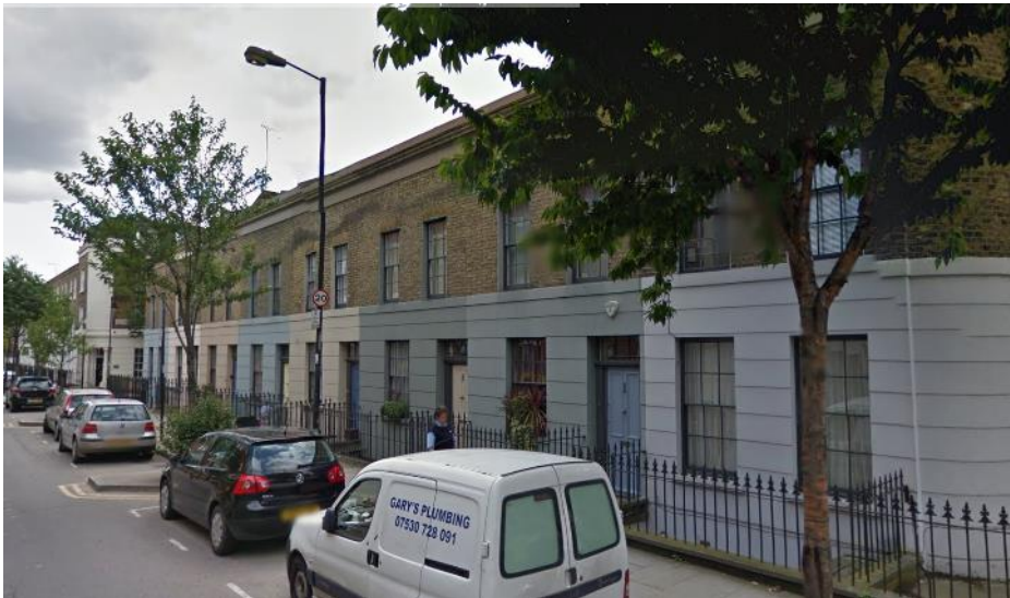
Image 1: Front elevation of the locally listed terrace at Wharfedale Road looking east
